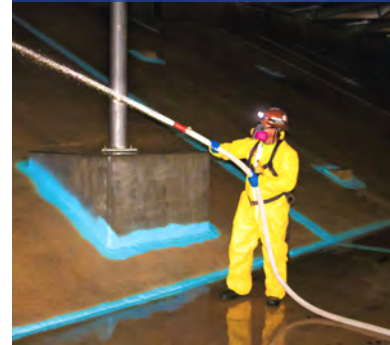
Crews thoroughly sanitize the interior of the reservoir to prepare for refill and water storage
