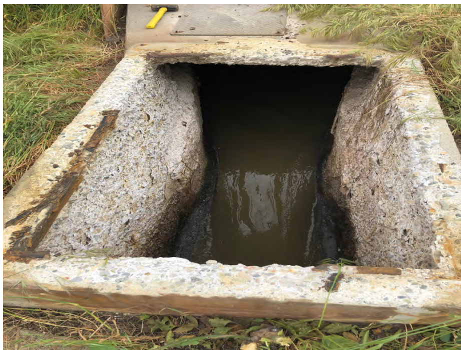
Figure 10-4: Concrete Structure on Pipeline 08700140860134
