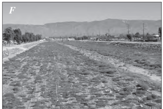
Warm Creek bypass channel, September 2004.
