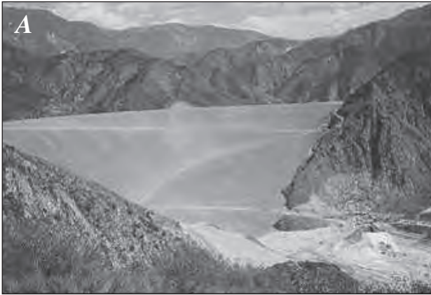
Seven Oaks Dam, April 1999. Photo courtesy of David Lovell, San Bernardino County.
