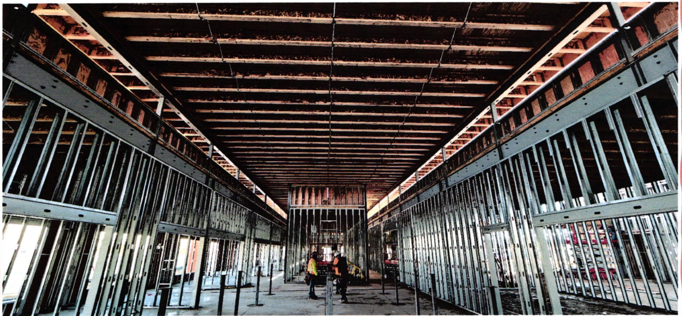
Rough Framing in the Engineering Area
