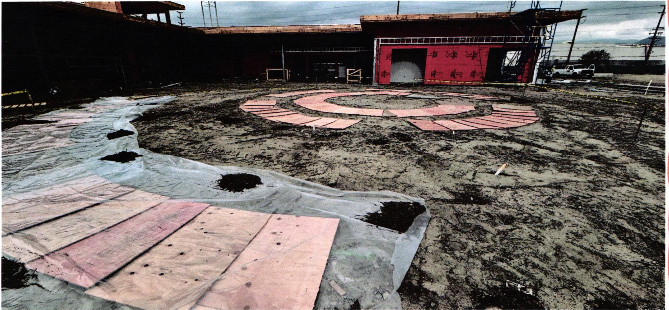
Protecting Excavations for Footings in Demonstration Garden
