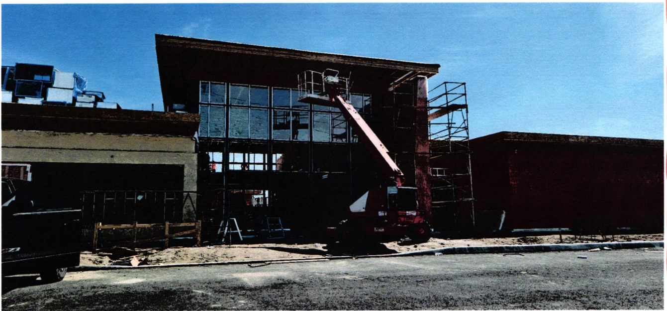
Placing Stucco and Glass at Front Lobby Exterior
