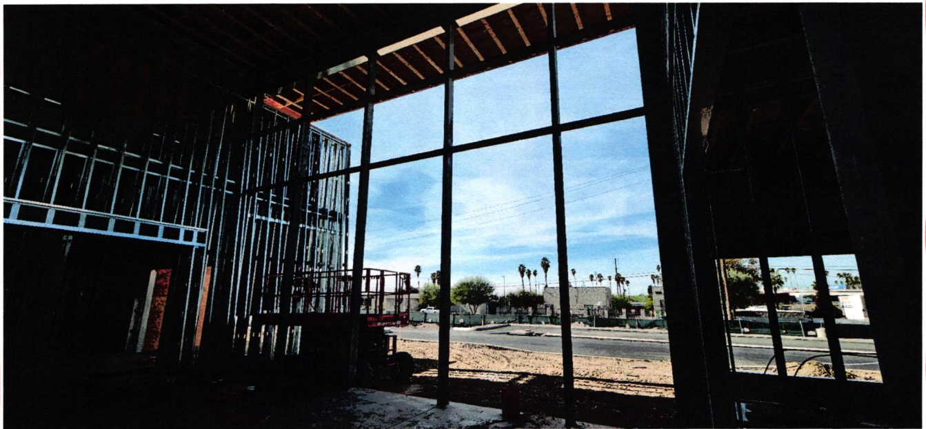
Rough Framing in Lobby Area
