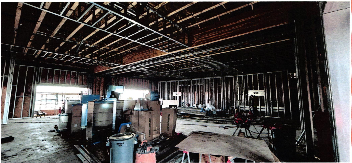
Interior Finishing of Water Board Room
