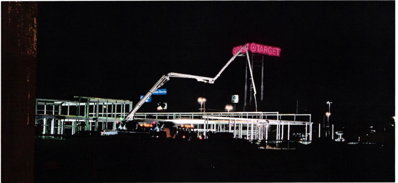
Pumping Cement in Early Morning Hours
