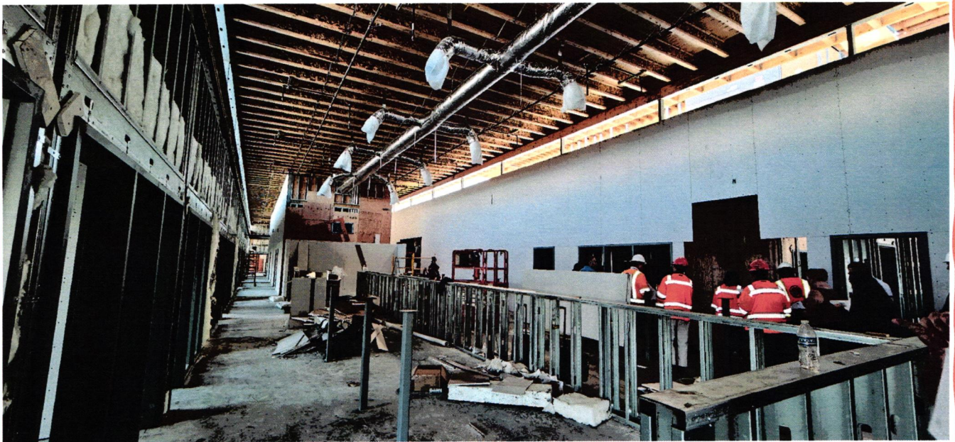
Interior Finishing of the Engineering Area
