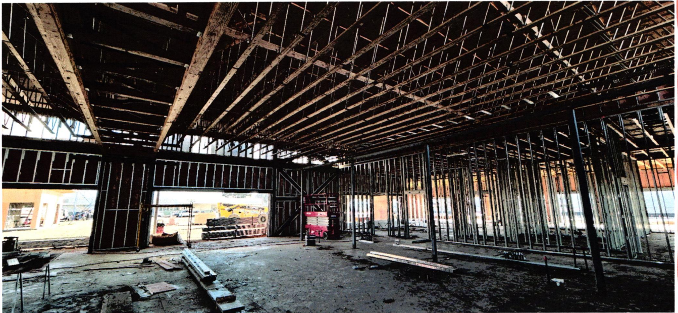
Rough Framing of Water Board Room
