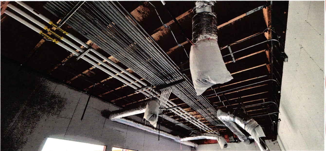
Rough Electrical, Plumbing, and HVAC Work Above Ceiling
