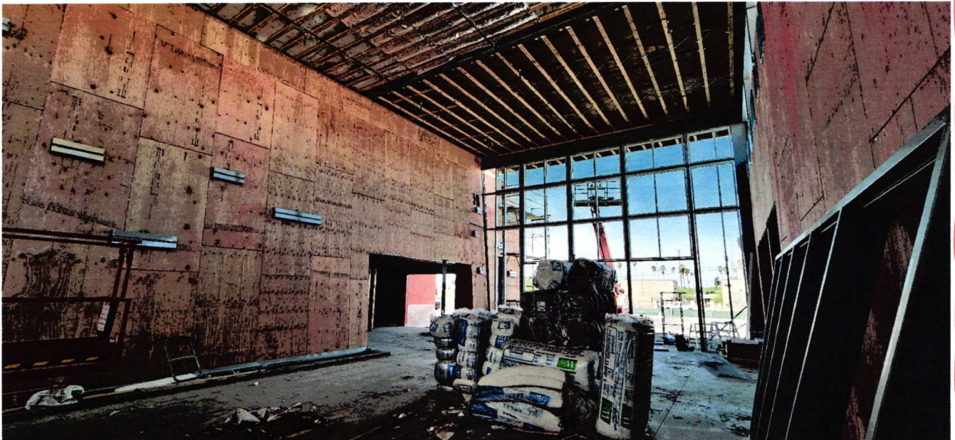
Interior Finishing of Lobby Area
