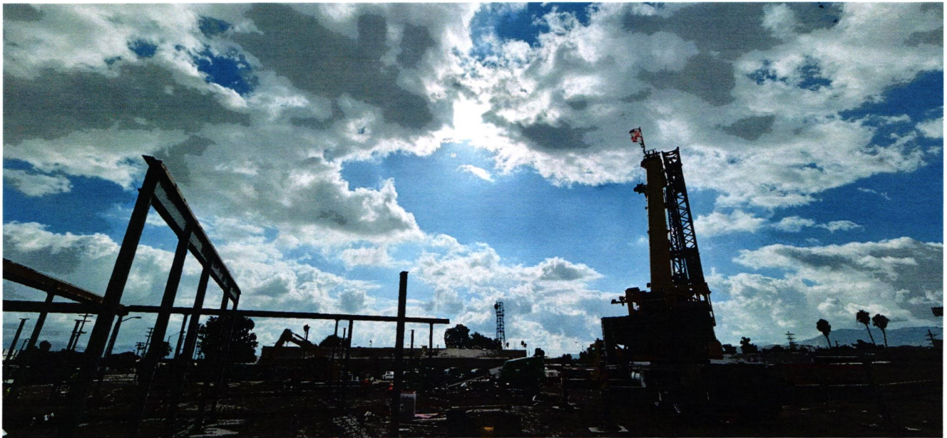
Installation of Structural Elements
