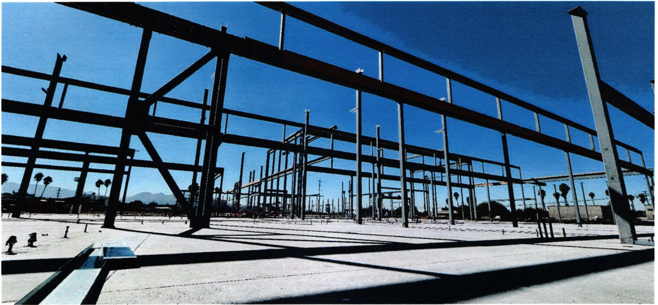
Foundation and Main Structural Components Completed
