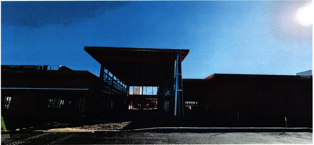
Rough Framing and Shear Panels of Front Lobby Exterior
