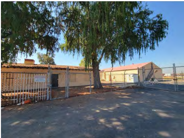
Southwest view of the building improvements.
