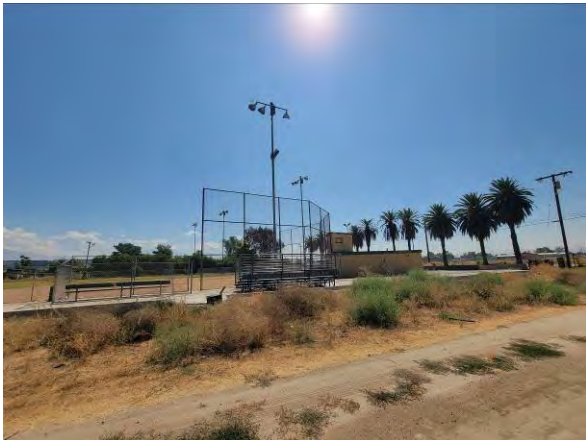
East view of the baseball field improvements.
