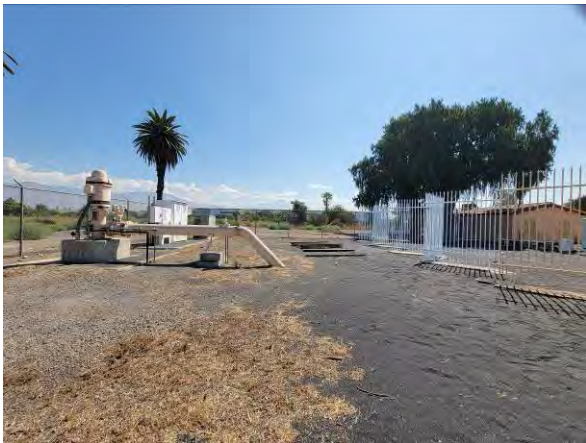
View of the well site.
