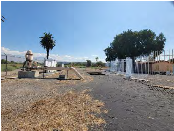
View of the well site.
