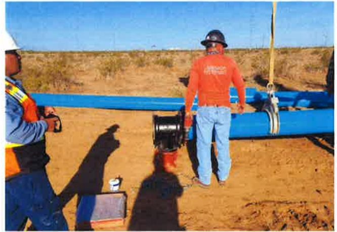
Adelanto Rd and Pansy Rd. Water and Sewer Project | City of Adelanto
