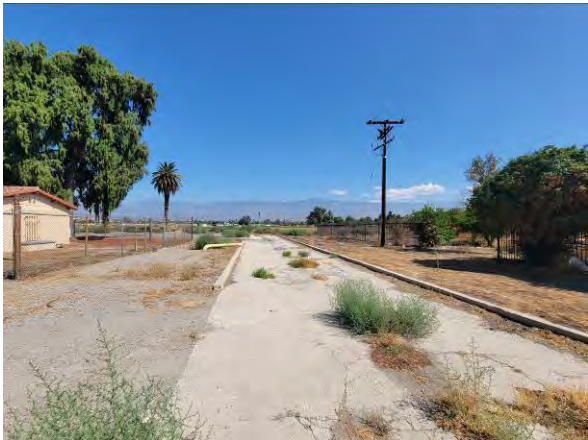
Northerly view of the east side of the property.
